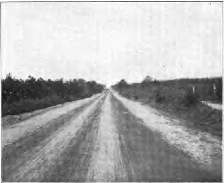
Corliss Avenue, Monmouth Co., after improvement.
